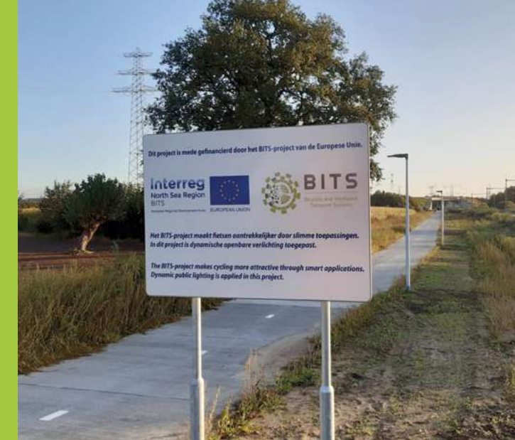
Figure 2.3: Dynamic lighting in Zwolle
