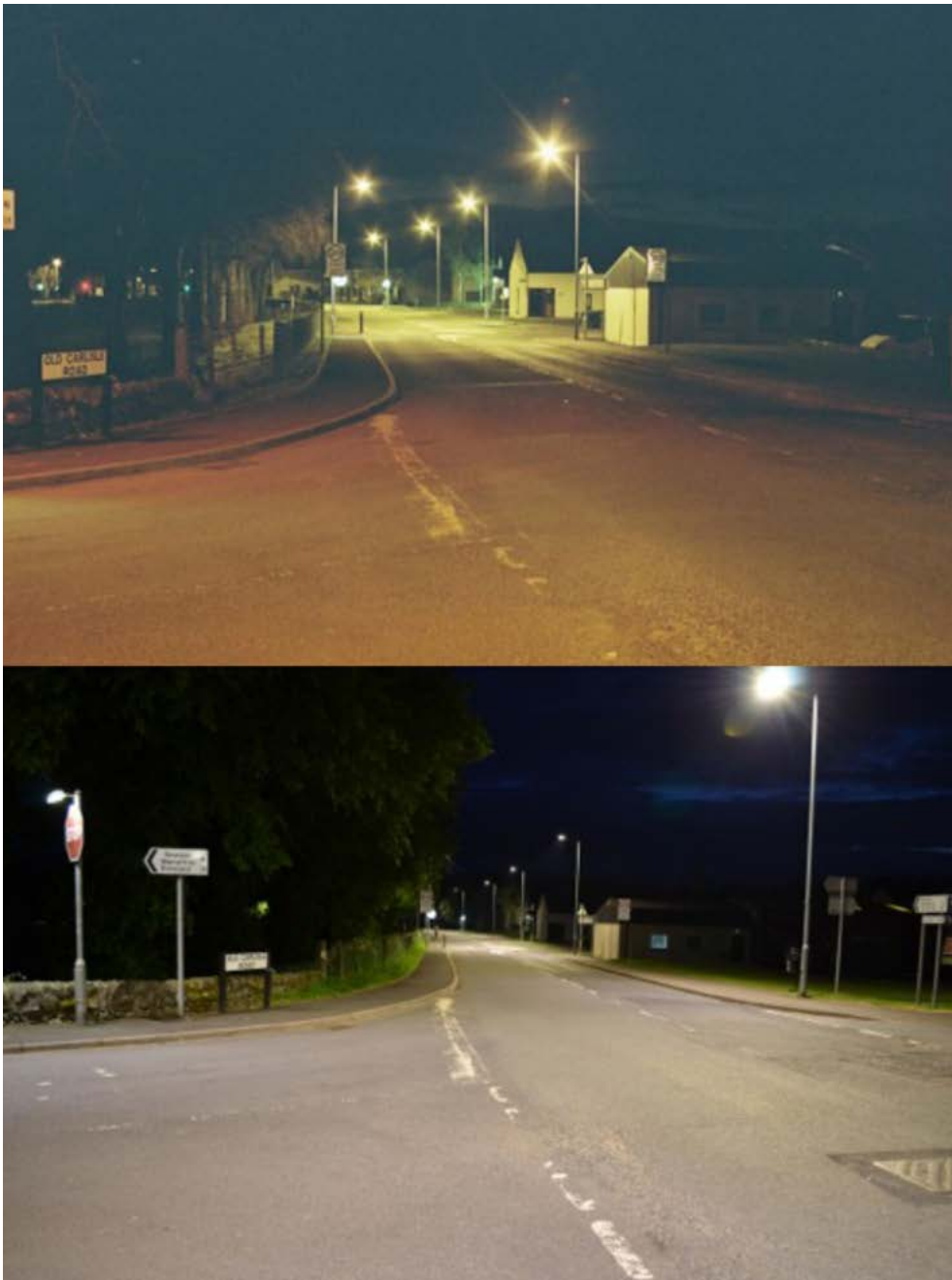
Figure 3.17. Views from The Holm, Moffat, UK, before and after retrofit. Source: IDA
