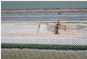
Section 1: The ecotoplayer on the Levvel blocs on the lower slope, existing of a roughened toplayer and 2 holes
