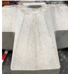
Section 1: The ecotoplayer on the Levvel blocs on the lower slope, existing of a roughened toplayer and 2 holes
