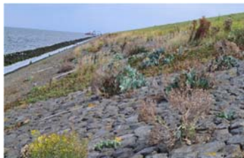
Section 1: The ecotoplayer on the Levvel blocs on the lower slope, existing of a roughened toplayer and 2 holes
