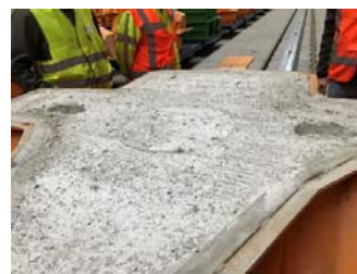
Section 1: The ecotoplayer on the Levvel blocs on the lower slope, existing of a roughened toplayer and 2 holes
