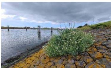
Section 1: The ecotoplayer on the Levvel blocs on the lower slope, existing of a roughened toplayer and 2 holes
