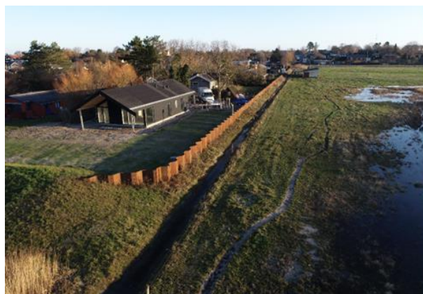
Figure 0.6 Installed sheet pile flood protection at Næsby strand
