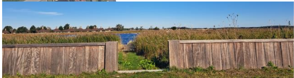
Figure 0.4 Installed vertical wood wall next to the N2000 area at Enø
