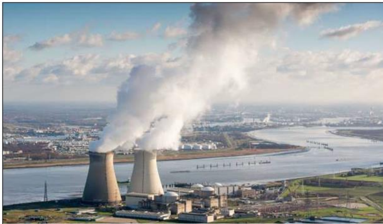
Doel Nuclear Power Plant
