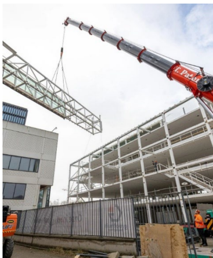
Figure 9: Disassembling temporary courthouse. (remountable construction: showcase temporary court in Amsterdam | cepezed, 2016)
