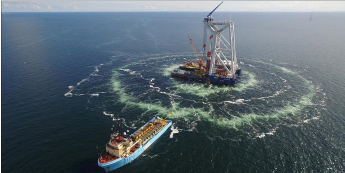
Figure 2. Use of a bubble screen to reduce effect of piling
